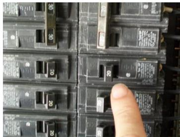
3. Push the breaker to the OFF position and back to the ON position. The breaker should appear the same as the remaining breakers.
